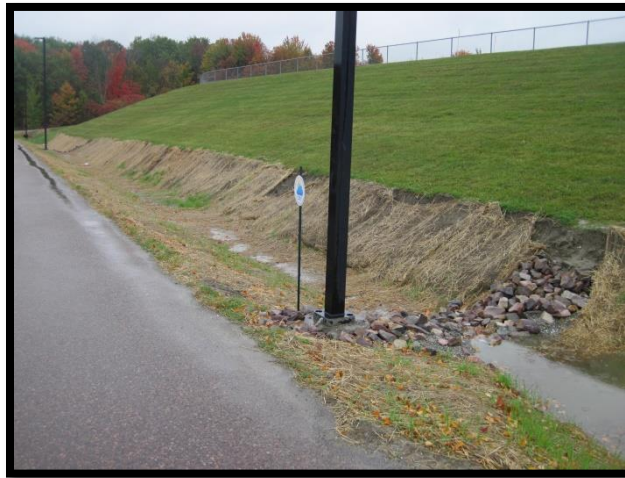
Completed bio-retention area at CVU, October 2020
