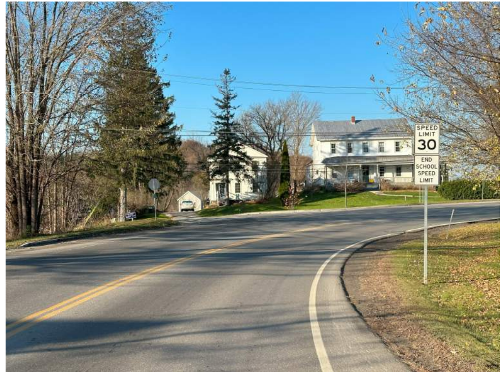
Westbound Approach to Intersection
