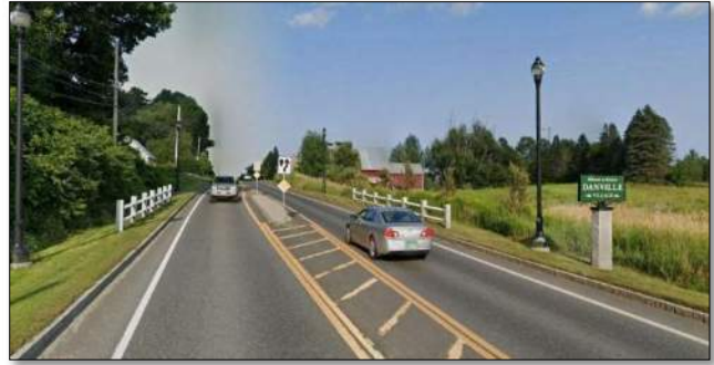
Gateway feature on US 2 in Danville, Vermont with median, split rail fencing, decorative lighting and a prominent sign. Raised median is five feet at its widest point.
