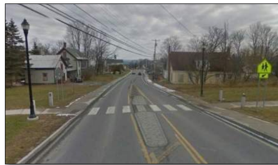
Flush median with contrasting stamped concrete and granite edging on US 2 in Danville, Vermont
