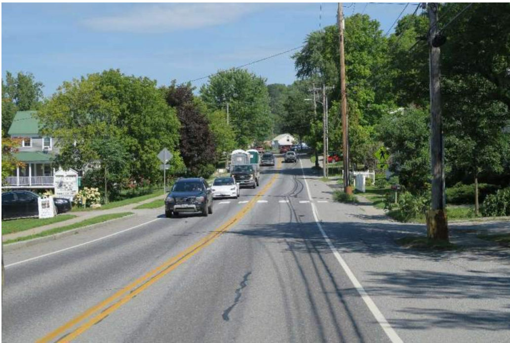
Photo 2. Northbound view on VT Route 116 by United Church of Hinesburg, taken south of the Church crosswalk on the east side of the street, looking north. Existing pedestrian warning sign partially obscured by tree and outside of drivers' field of view.
