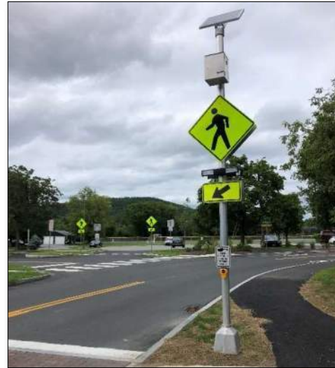
Example of RRFB with push button activated flashing beacon powered by solar panel.
