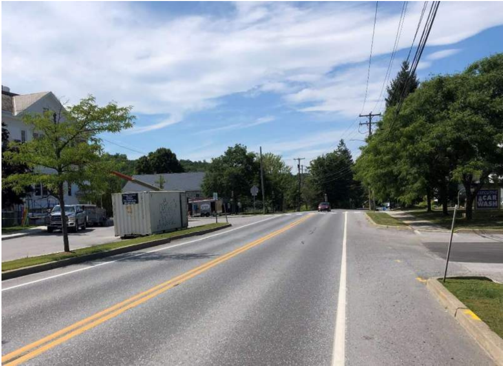
Photo 5. Westbound view of VT Route 116 taken stopping sight distance in front of Hinesburg Community school. Note that pedestrian crossing warning sign obstructed by tree foliage.
