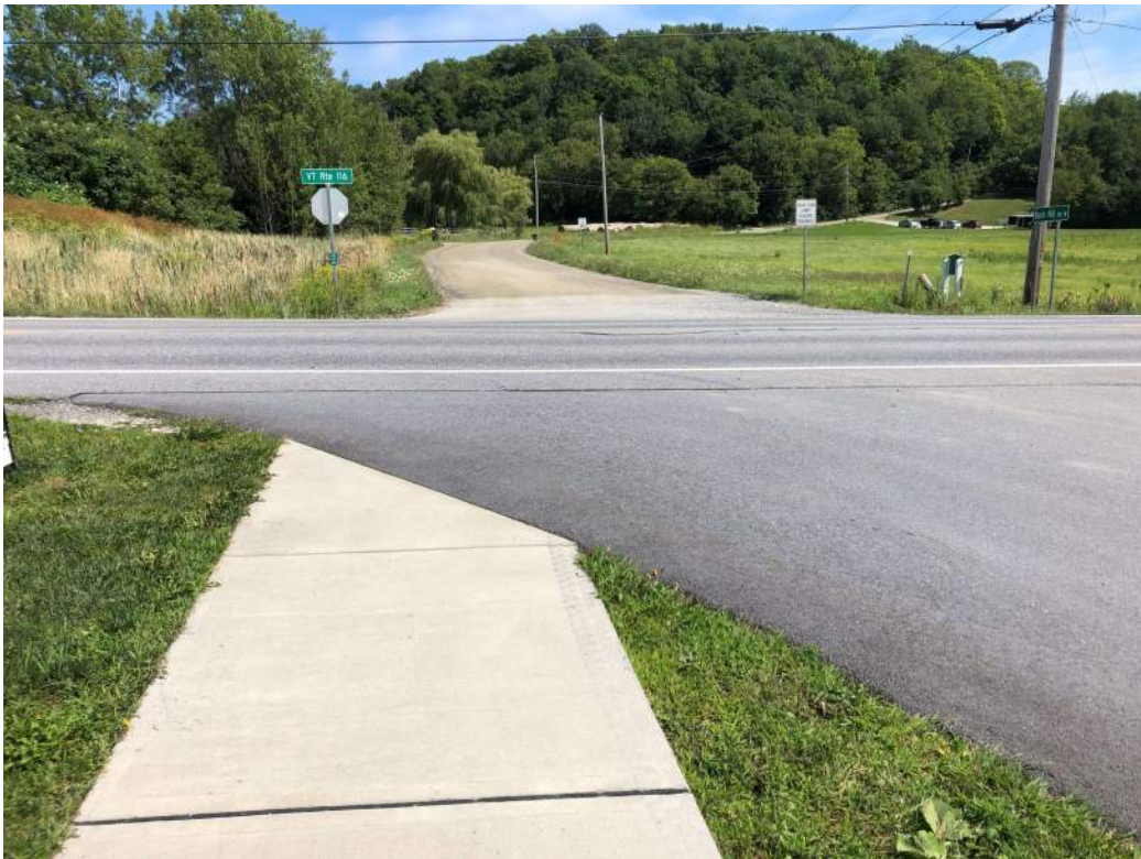
Photo 10. Eastbound photo taken on Clinton St. (newly developed road to housing), just east of its intersection with VT Route 116 showing the newly installed sidewalk connecting the housing development to VT Route 116.
