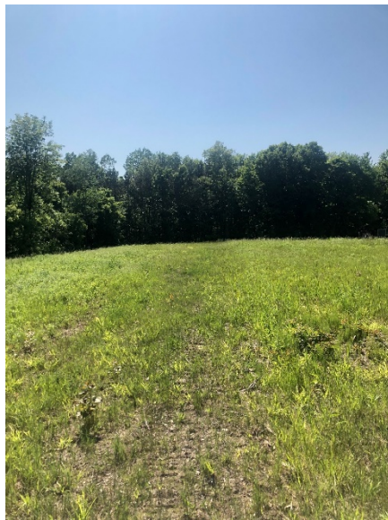
Photograph #2: View of landfill cover- 5/30/2023.
