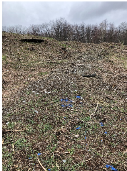
Photograph #4: View of exposed debris on eastern slope, shown on Figure 2 as area requiring topsoil.
