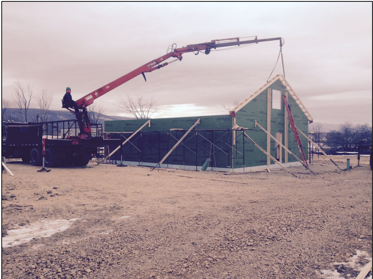
Trusses are being added to the Water Treatment Facility Building - January 26, 2016
