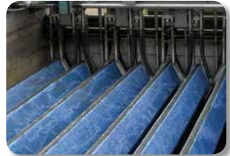
An AquaDiamond® filter with Microfiber cloth polishes phosphorus to < 0.1 mg/l.
