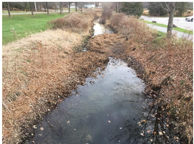
Patrick Brook Canal at a section with only stagnant water from local runoff or remnants of flood waters entering at diversion structure (no flowage when picture was taken). Sediments accumulating in the canal would otherwise have enter the lower reach and contributed to the beneficial re-meandering and channel evolution currently underway.
