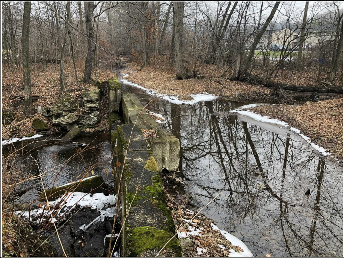
Photo #1 - Patrick Brook "dam" looking north
