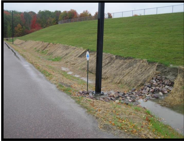
Completed bio-retention area at CVU, October 2020
