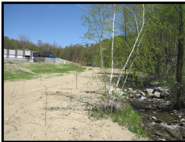
Completed Beecher Brook floodplain restoration at Hinesburg Town Garage, May 2020
